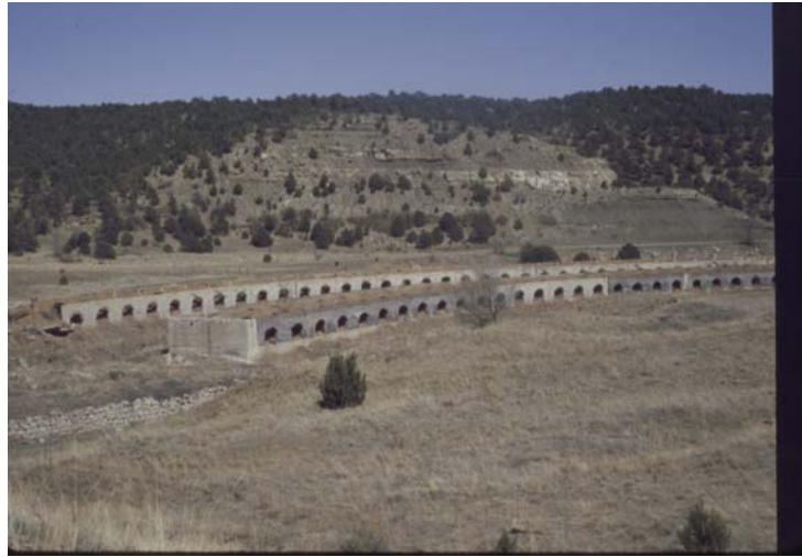
Coke ovens at Cokedale
